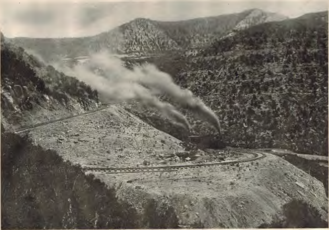
Moro Beagle Curve, One Mile from Atchee; 66 Degrees on a Grade of 7½ Per Cent
